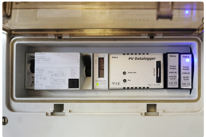
Figure 1: The finished energy logger with meter and power supply unit, installed in a small plastic distributor.
