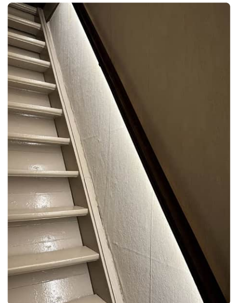
Figure 1: The author used the circuit described in this article to provide safe lighting for a staircase. Under no circumstances may the light switch off when someone is on the stairs. The LED strip is mounted under the stair railing and illuminates the steps. The sensor is located at the top of the staircase, so all of the steps are within the radar's range.
