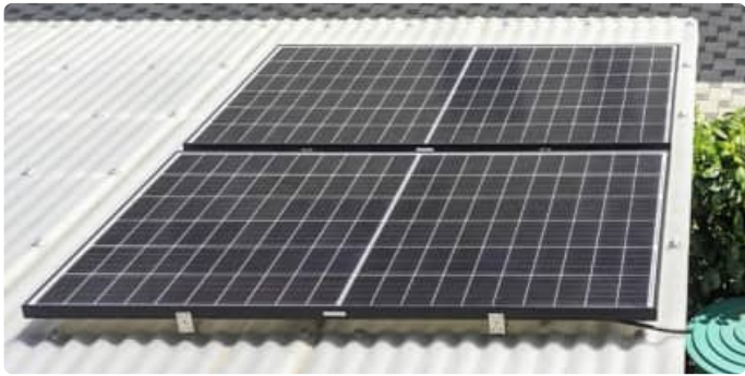
Figure 2: The two 330 Wp panels of my first balcony power plant on a canopy.
