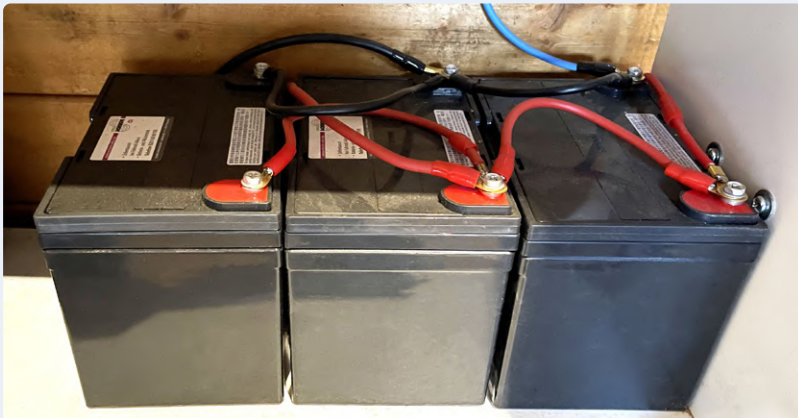
Figure 3: Three 12 V lead gel batteries, each rated at 36 Ah, are wired in parallel to act as energy storage in Klaus' shed.
