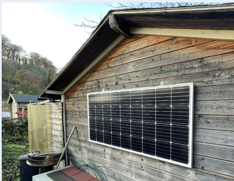
Figure 2: The 12 V solar panel mounted vertically on the wall of Klaus' shed. It has an output rating of 180 Wp.
